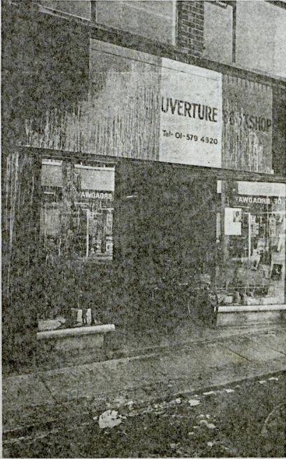
The wrecked facade of Bogle L'Overture, a typically cluttered, quiet bookshop which supplies many multi-cultural books to schools throughout the borough.
